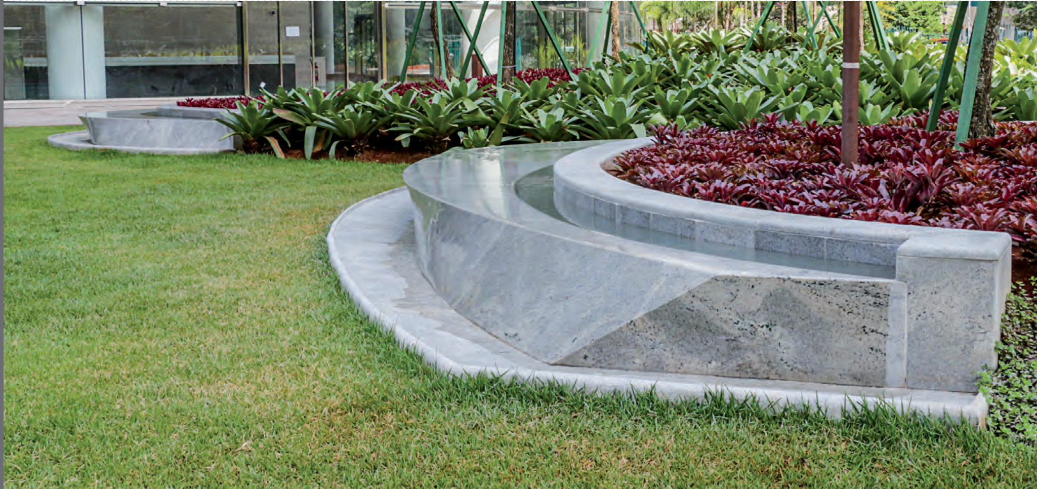
HIMALAYA · MAGNIFIC GOLD SÃO PAULO CORPORATE TOWERS PROJECT BY PELLI CLARKE PELLI LOCAL LOCATION SÃO PAULO
