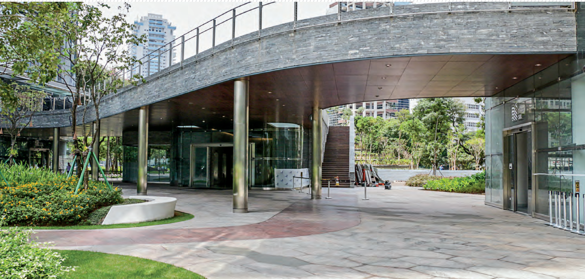
HIMALAYA • MAGNIFIC GOLD SÃO PAULO CORPORATE TOWERS PROJECT BY PELLI CLARKE PELLI LOCAL LOCATION SÃO PAULO
